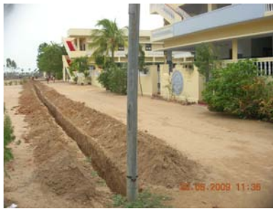
Bore hole and pipe trench
